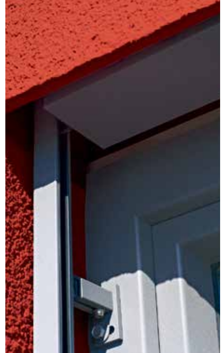
Headboxes or other custom enclosures house the blinds when retracted, providing protection from high winds and other severe conditions.
