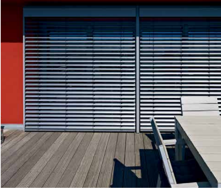
Moving slats to the open position during wind allows pressure to equalize.
