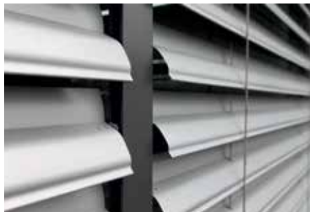
Moving slats to the open position during wind allows pressure to equalize.
