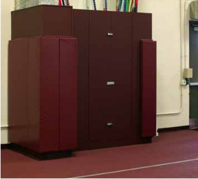
Everything is a potential hazard, and should be padded. Even corners—including all outside corners—and columns should be padded.
