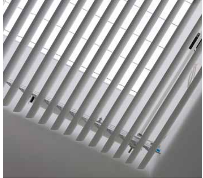
Rack Arm systems are a highly effective shading solution for skylights.
