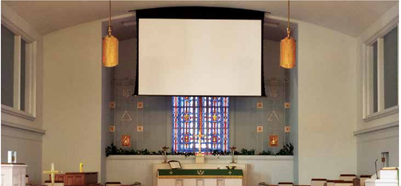
Ceiling-recessed projection screens are a simple solution to hiding a screen when not in use. There are several different models depending on the solution required.
