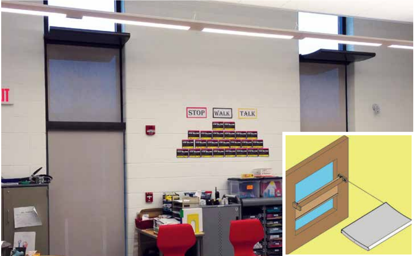
Photo: Flexwave Light Shelf & Motorized FlexShades. Dealer: Shadeology. Photographer: Al Marx of Shadeology. Insert: This close-up drawing shows how the shade bracket is integrated with the FlexWave bracket on an inside mount.
