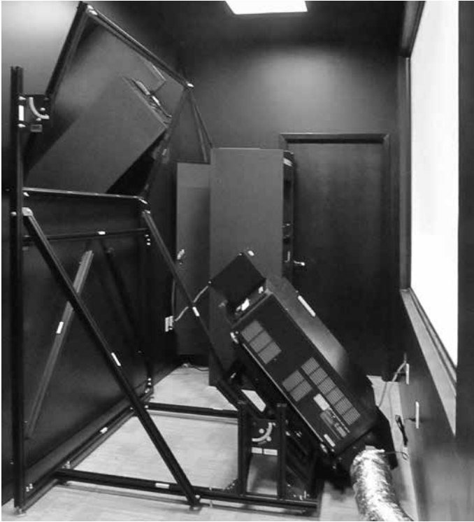
RPX/Precision mirror and support structure, Dealer: Vistacom, Allentown, Pennsylvania Client: Alvin H. Butz, Inc., Photography by: Alvin H. Butz, Inc.
