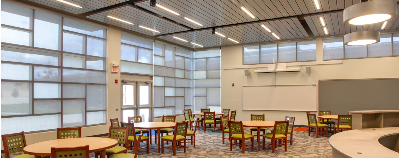
Motorized Shades using Sun Solutions Controls, Alcalde Elementary School, Espanola, NM Architect: FBT Architects. Photography: Matt Oberer, Matt O Photo Albuquerque, NM
