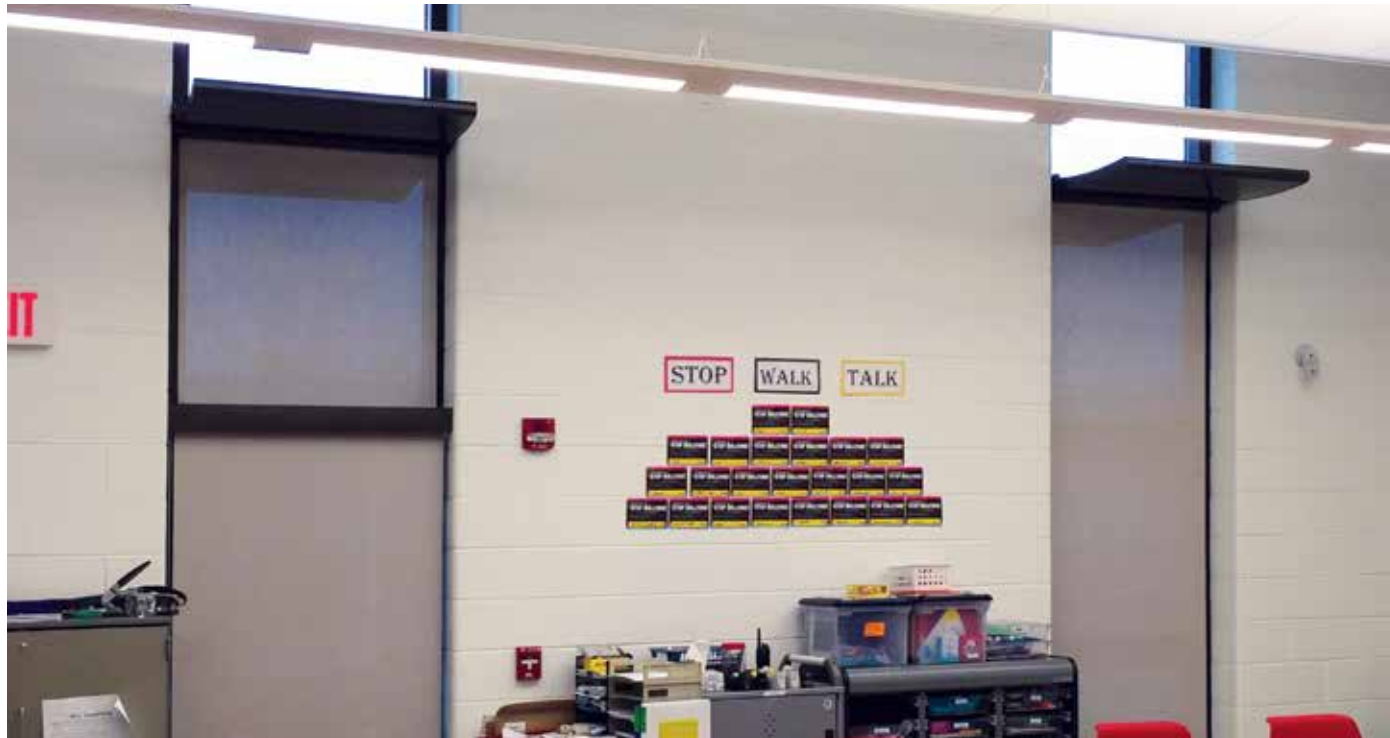
FlexWave™ Light Shelf and Motorized FlexShades®, Glen Elyn Churchill Elementary School, Chicago, IL., Dealer: Shadeology., Photography: Shadeology
