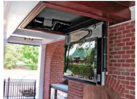
Custom Monitor lift, Chile Banco left, other custom work above.
