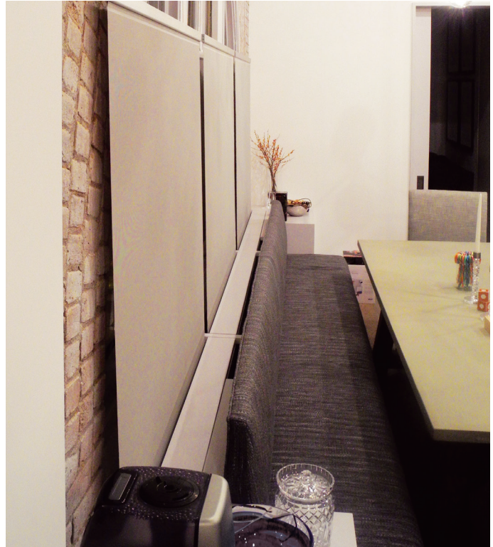
A side view showing the custom millwork behind which the operating system and rollers were hidden, making the unit invisible when retracted.
