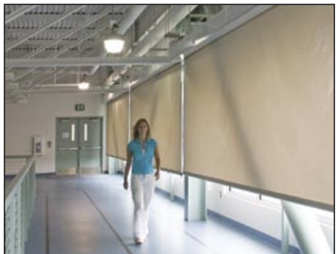
Colossal FlexShades at Wasilla (AK) Multi-Use Sports Complex. Architect: Kumin Associates, Anchorage, AK. Installation: Carberry & Associates. Photography: © 2005 Robert Baker, North Star Multimedia, Wasilla, AK.
