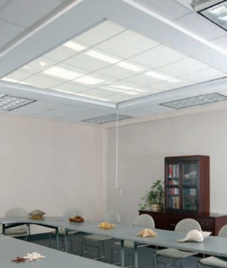
Skylight FlexShade with "E" Screen 5% at Lawrence North High School. Installation: SPD Textile & Drapery, Inc. Photography: © Brian Bookwalter. All of Indianapolis, IN. Shown closed above, partially open below.
