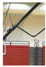
Securely lock backstop into playing position, the TF-20J Basketball Backstop features the exclusive "hammer lock"—a stem-weight actuated positive latch. Stem weight eliminates the need for supplemental retractors or stretch cords. Includes integral cable retraction system. Backstops are custom designed so the lateral sway brace intersects the main mast at approximately 54" (137 cm) above the goal and 18" (46 cm) above the backboard; to ensure maximum rigidity.
