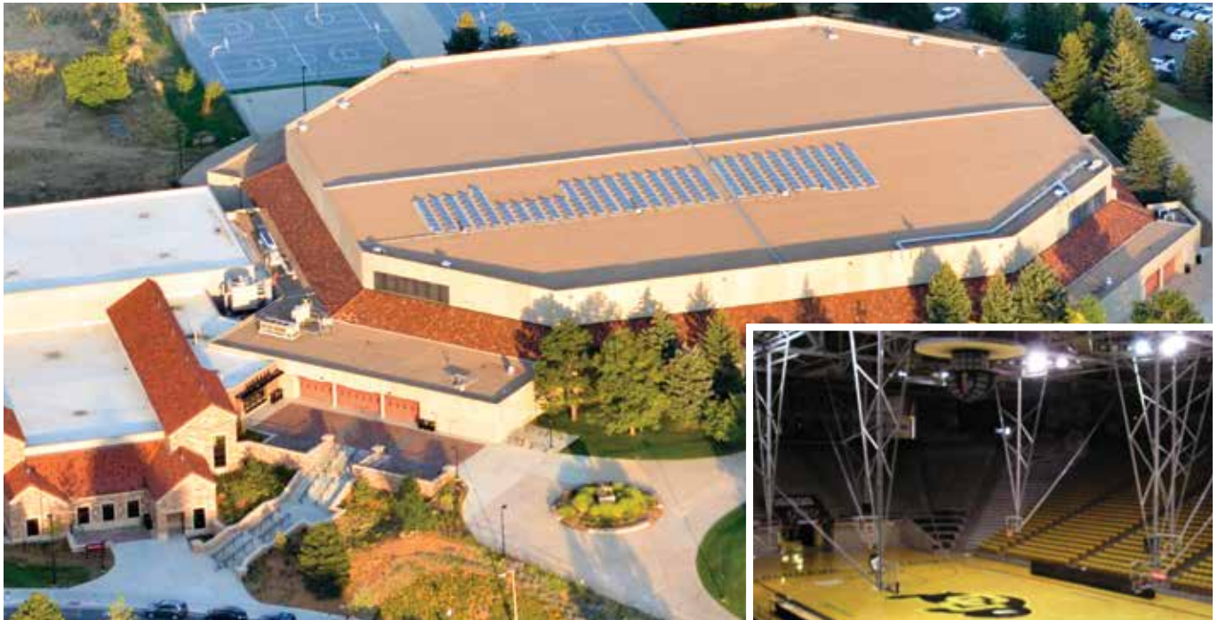
Exterior view of the Coors Events Center, home of the University of Colorado Buffaloes. Photo courtesy University of Colorado. Inside the renovated facility, Draper's EZ-Fold TB-25B rear folding backstops are ready for action!
