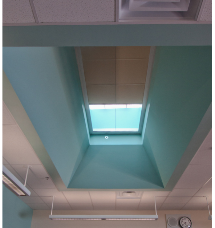
Skylight FlexShade, ABOVE: Wherry Elementary in Albuquerque, NM Photography: Matt Oberer, Matt O Photo, Albuquerque, NM
